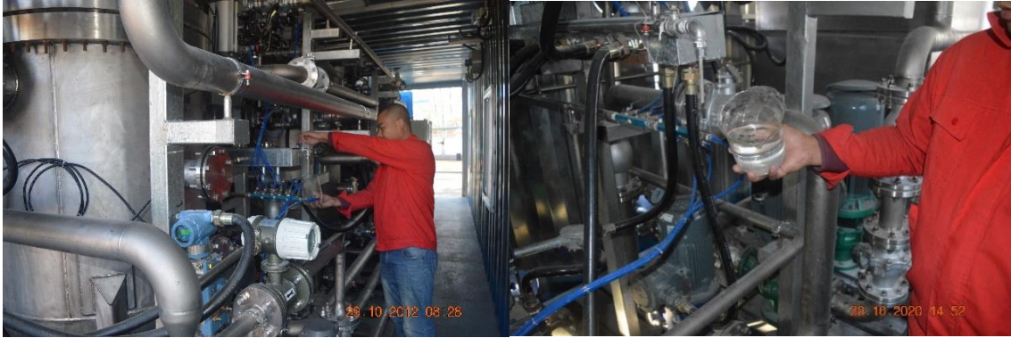
Figure 11: Dajing China: Operators taking samples on 25 m 3 /hr Replaceable Skin Layer Membrane.
