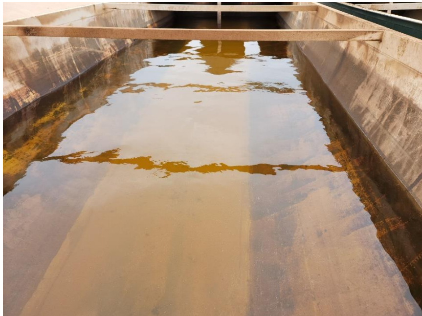
Figure 20: Frack tank storing Permeate from the treatment of Produced water by Replaceable skin layer membranes.
