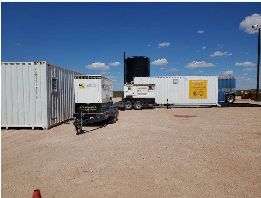
Figure 21 Setting up Replaceable skin layer membranes Sea Container unit at SWD Facility – Barstow TX
