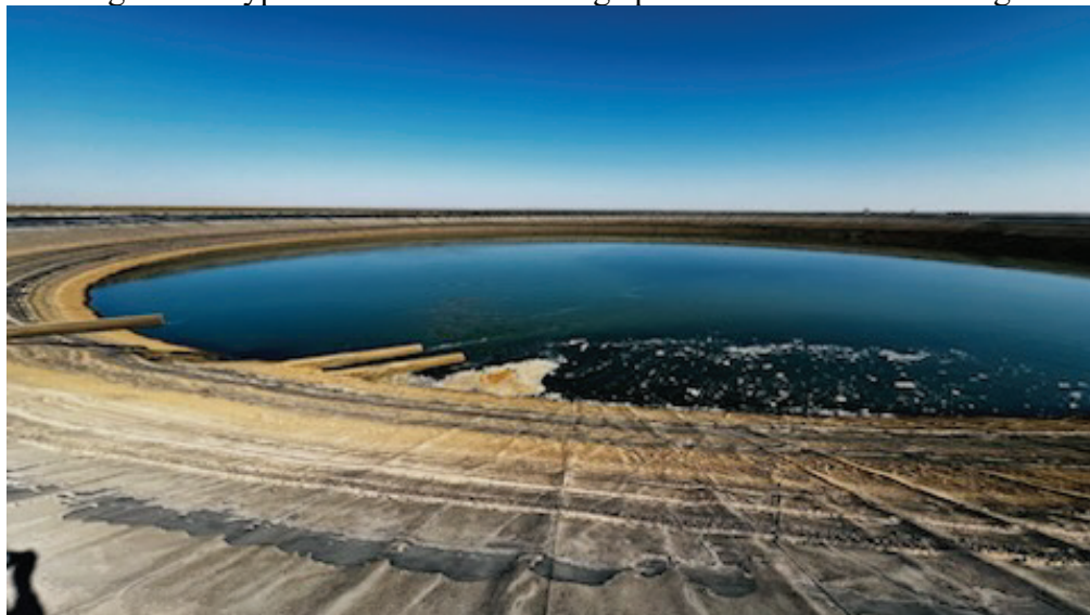
Figure 28 Typical treated water storage pond with iron based sludge
