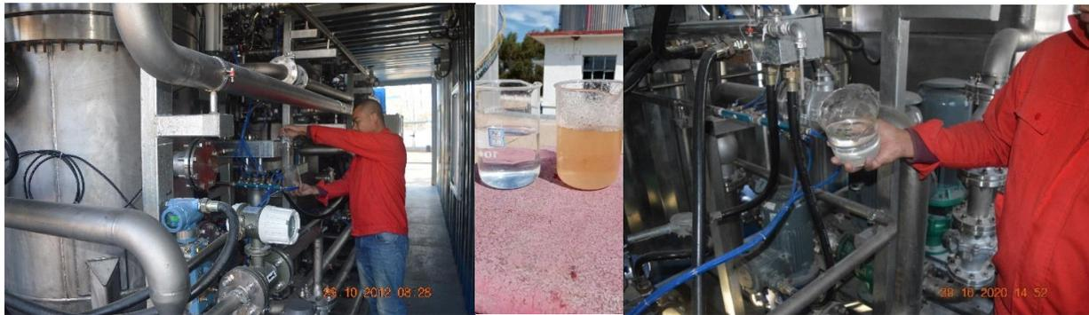
Left- Operator taking sample of raw water- Two Membrane Housings 12.5 m<sup>3</sup>/hr each
